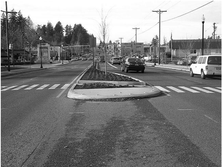
FIGURE 28: PEDESTRIAN REFUGE WITH "NOSE" CREDIT: KIMLEY-HORN AND ASSOCIATES, INC.
